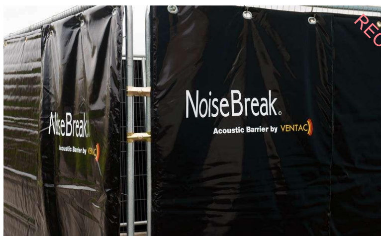
Figure 9-9: Temporary construction noise barrier © Ventac.
