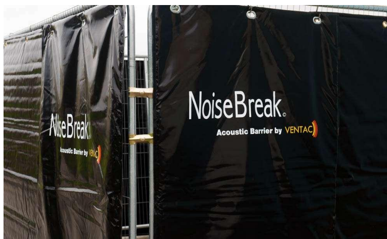
Figure 16-4: Temporary construction noise barrier © Ventac
